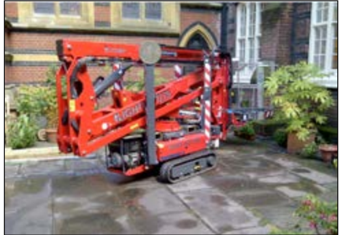
The Cherry Picker arrives at All Saints for the Lighting and Electrical Renewal project to get underway, October 2014.
