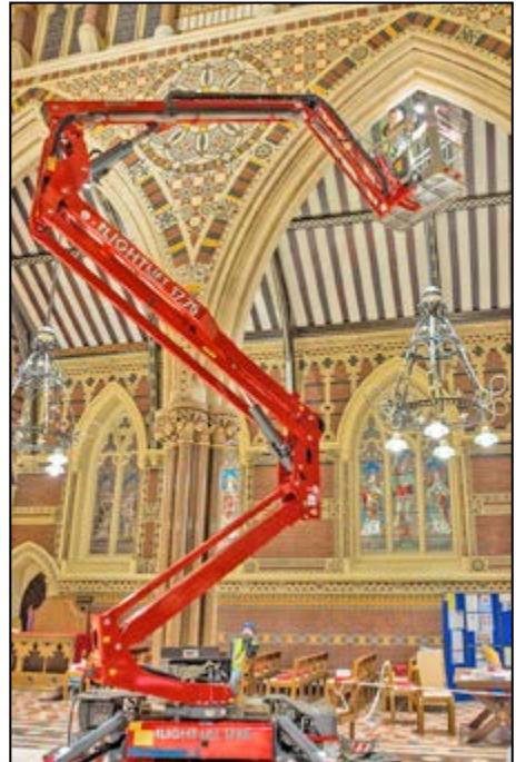
Final focusing of the new Church lighting for Christ the King
